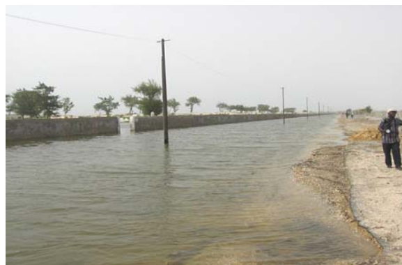
Floods in Saint Louis – ENDA Rup 2006 report
