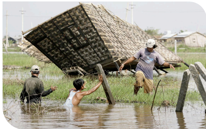
People repair a fence damaged by Cyclone Nargis on a road near Yangon, May 2008. Photo: REUTERS/Stringer.
