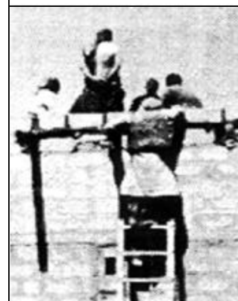
Training of builders in hazard-resistant construction techniques is best carried out through practical exercises and advice on-site.
