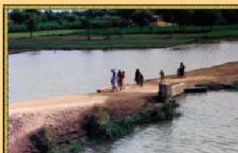
Culvert providing protection from floods and mobility to villagers during the monsoons
