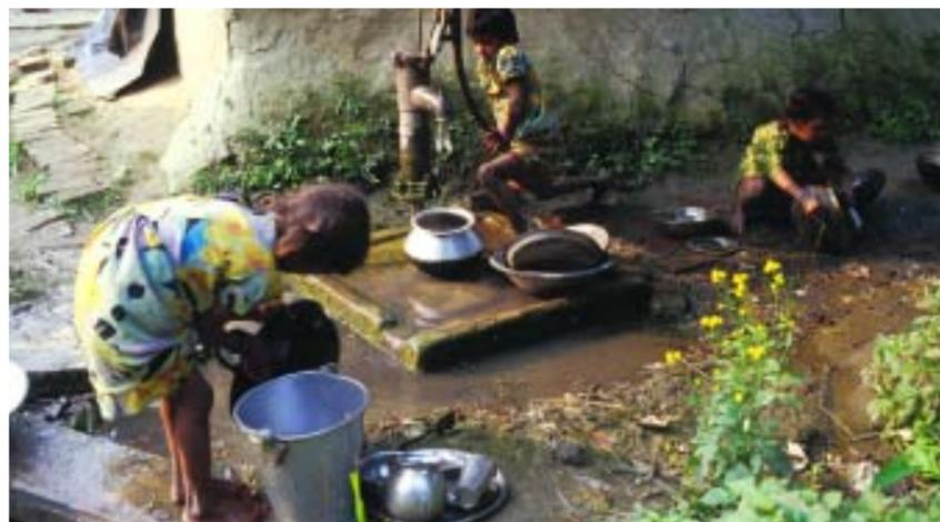
Low-lying hand pumps are rendered useless during flooding because they are submerged.
