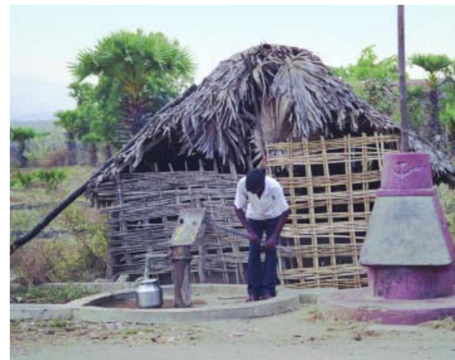
Low-lying hand pumps can be rendered useless in times of flood, and many do not draw water in times of drought.
