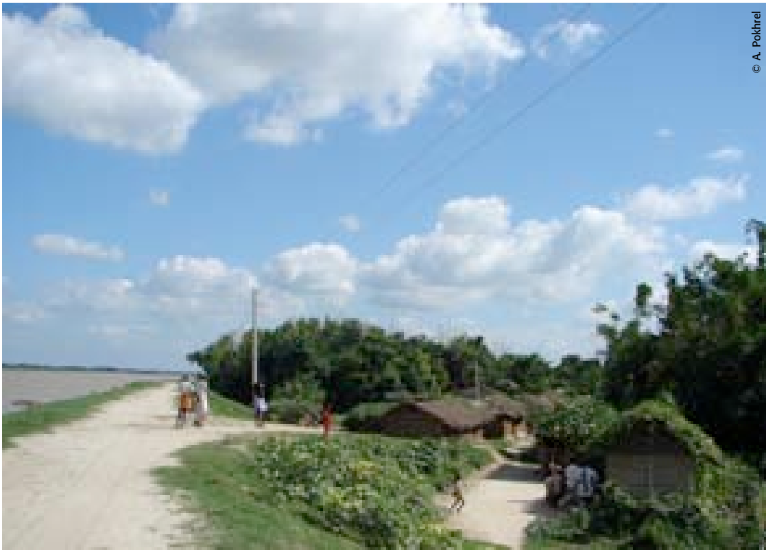
Embankment along Bagmati River at Brahmapuri, Rautahat District, Nepal.
