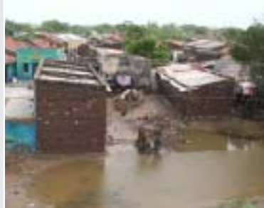
Rubble and mud after receded water, Jamnagar, Gujarat.
