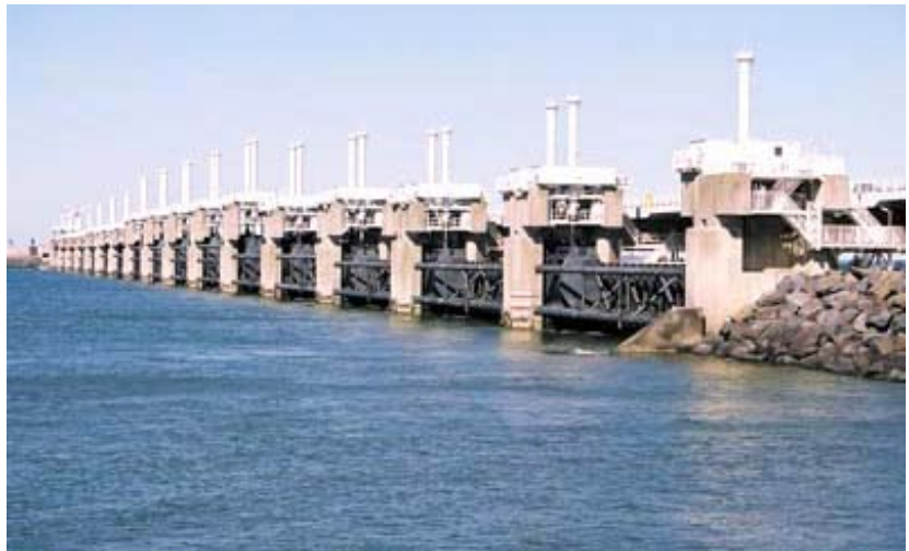
A Part of the Deltawerken; a dam with openings that can be closed during a storm surge. Source: margriethof.nl
